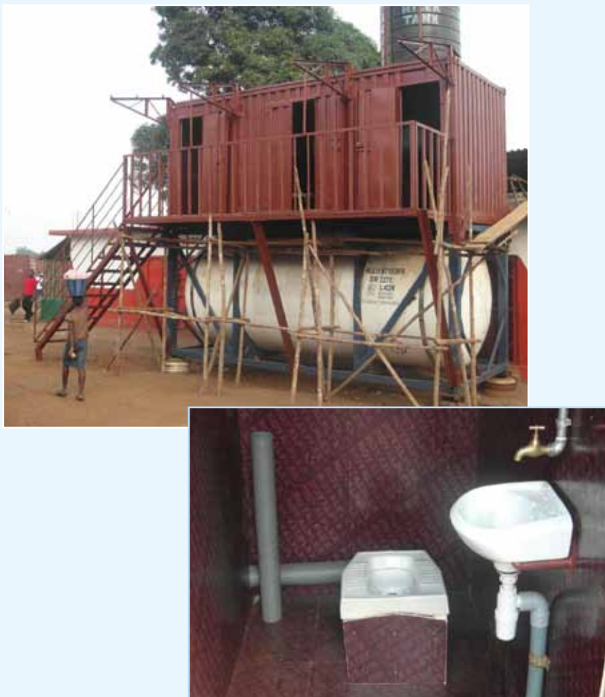
Figure 4.17 Large capacity modular and multi-functional transfer station (top), and sanitation facility (bottom) (photo: GOAL).
