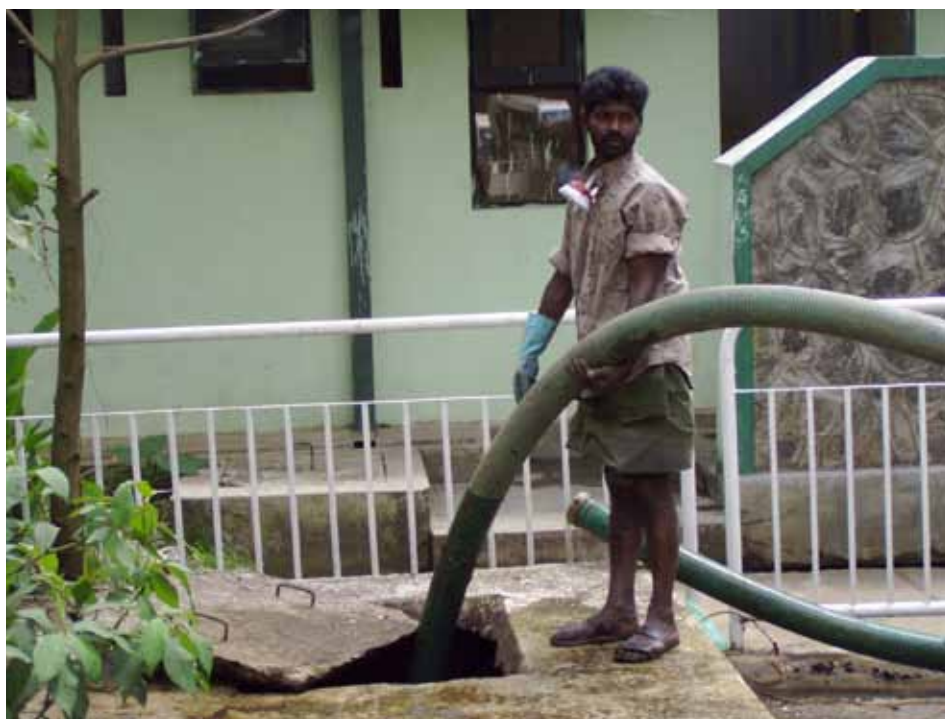
Figure 4.1 Emptying operation of faecal sludge from a septic tank using vacuum equipment. Job safety would be improved by better protective equipment (photo: David M. Robbins).
